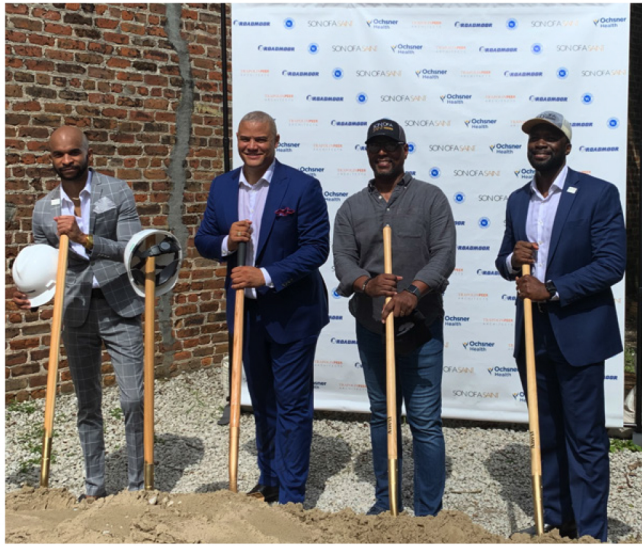
Elliot Hutchinson, Bivian "Sonny" Lee, Theo Sanders and Ola Adegboye at the groundbreaking for the new Son of a Saint center
